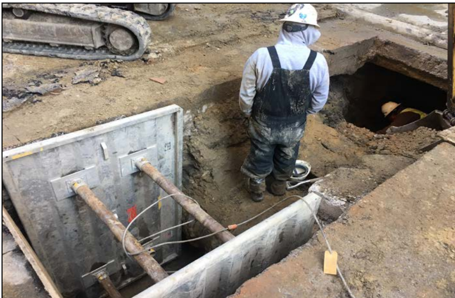
Photo 3: View facing northwest of excavation on Illinois Street (sewer runs underneath 3 foot water main worker is standing on)
