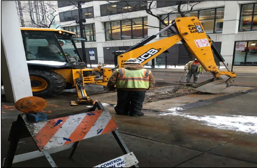
Photo 1: View facing south of excavating above sewer main on Illinois Street
