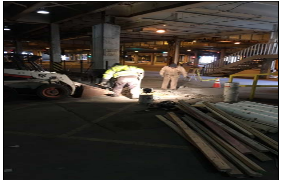
Photo 4: View showing forms for concrete pour.
