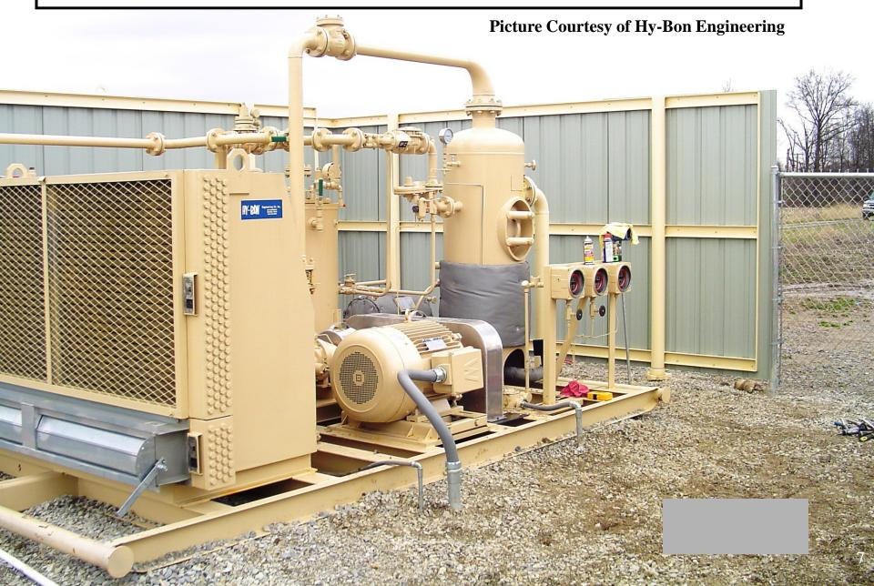
Rotary Screw compressors were used due to the wet nature of this gas stream. Filters are used before the skid to remove iron sulfide, then a scrubber vessel and automated liquid transfer system on skid to handle the liquids which are common in this application.
