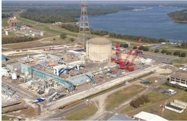
Waterford 3, St. Charles Parish
