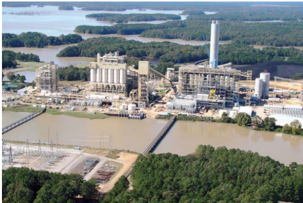
Brame Energy Center (Rodemacher)
