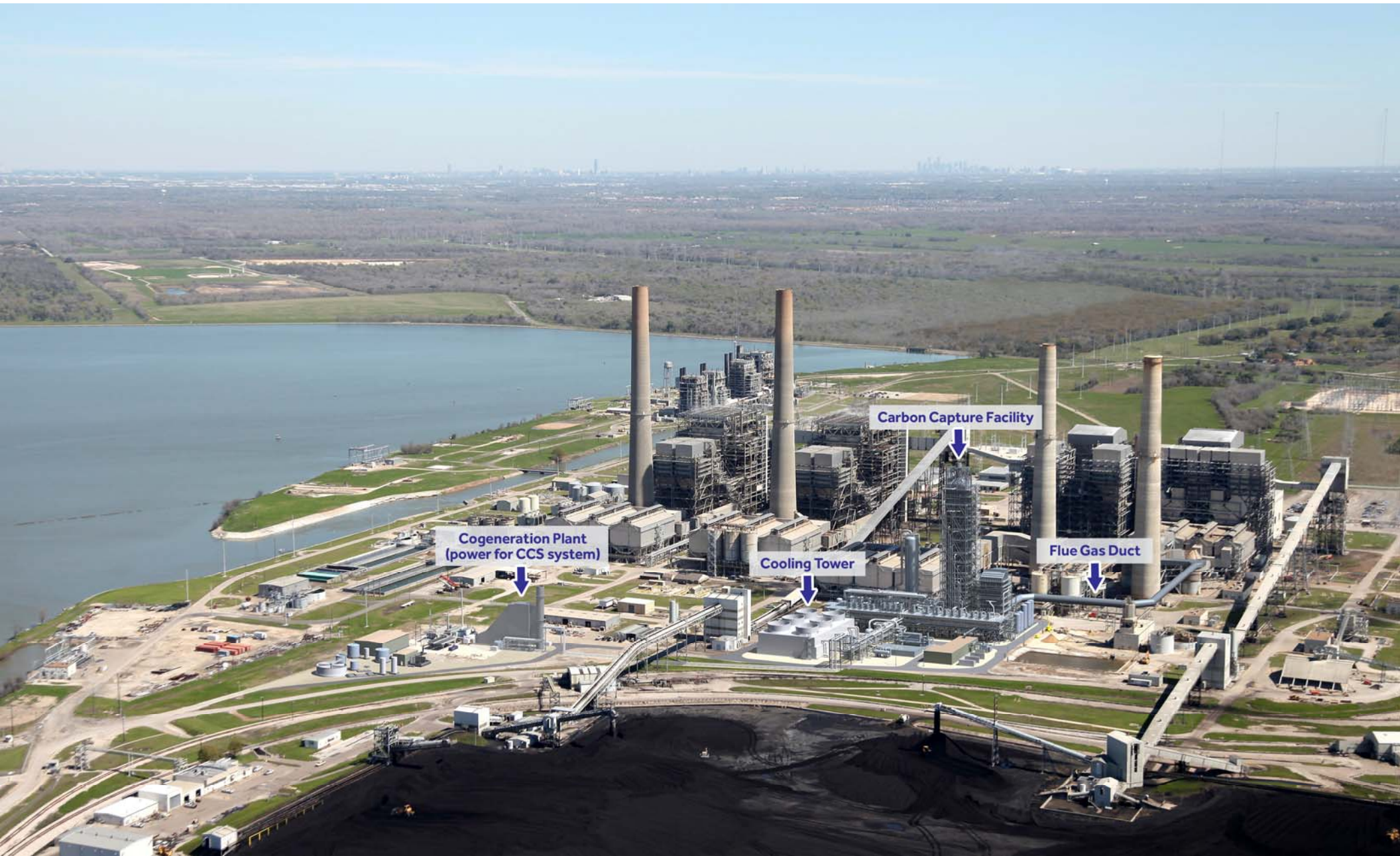
W.A. Parish Power Plant in Thompsons TX Proposed Carbon Capture Facility and Cogeneration Plant for the Carbon Capture System
