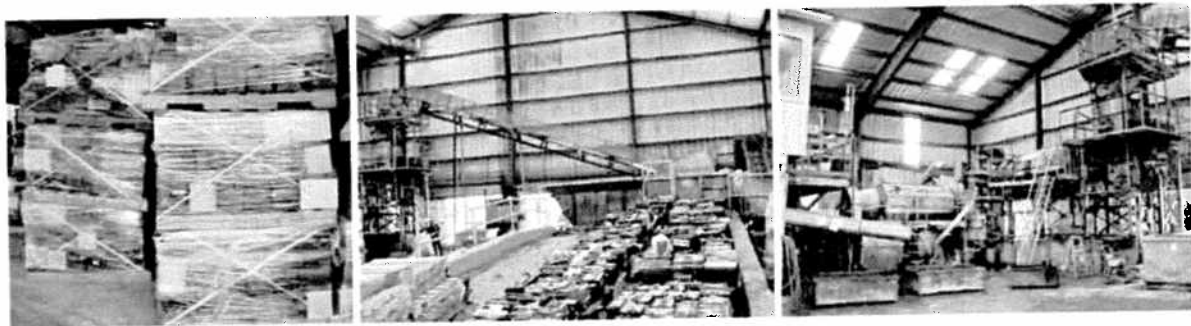
Figure 6. Received lead batteries, staging and conveyance, hammer mill and wet screening.
