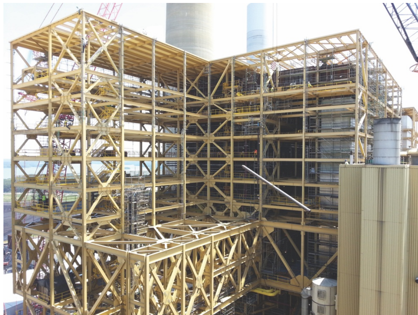
Selective Catalytic Reduction system support steel
