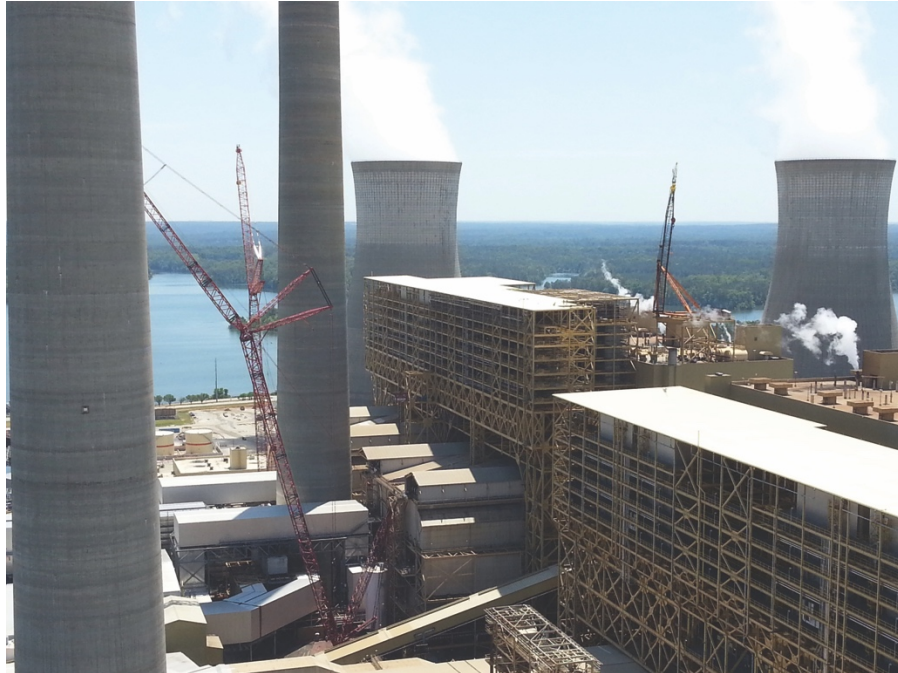
Units 1 – 4 Selective Catalytic Reduction systems
