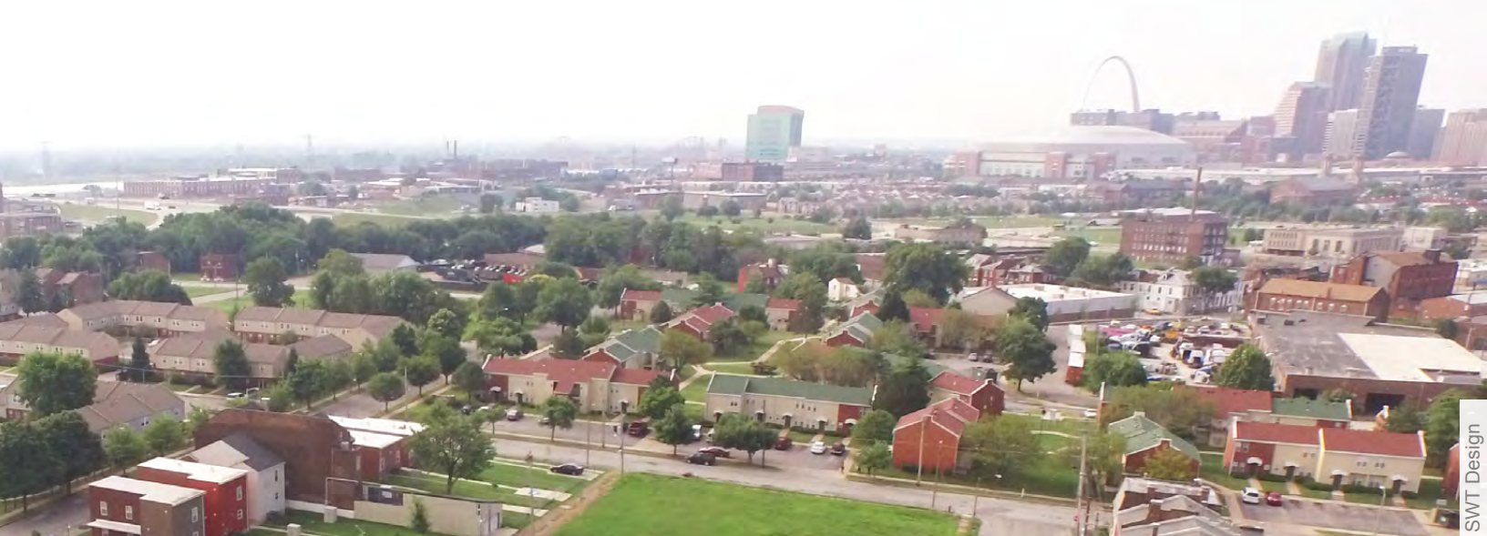
Figure 61 The Murphy Blair Gardens apartment complex, seen in the foreground, houses 114 HUD-managed Section 8 assisted living units. HUD has had major contributions to date to provide residents with affordable housing.
