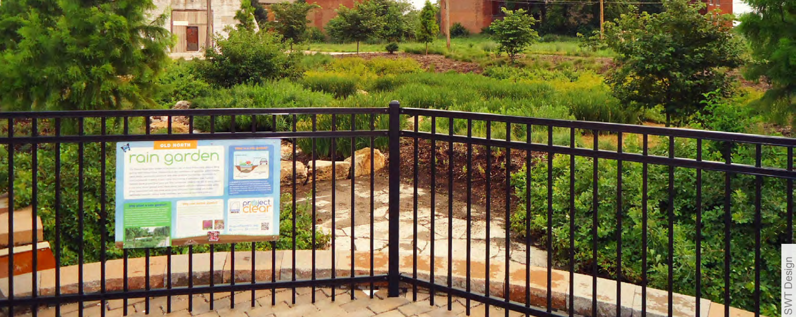
Figure 60 This Metropolitan Sewer District demonstration rain garden on the northeast corner of Clinton Street and North 14th Street manages runoff and educates residents and visitors about rain gardens.
