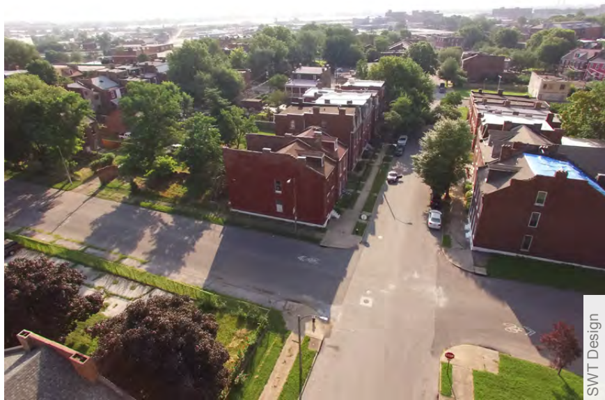
Figure 52 Existing condition, looking east toward the Mississippi River.
