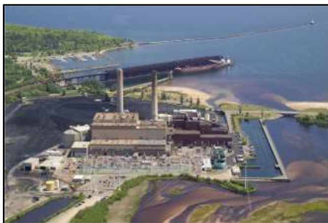
Figure 1. Presque Isle Power Plant
