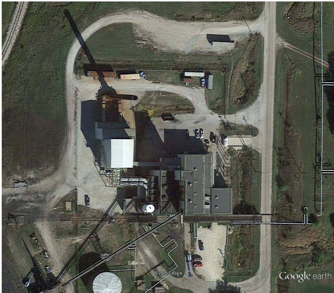
Figure 3-3 . Iowa Army Ammunition Plant boiler.
