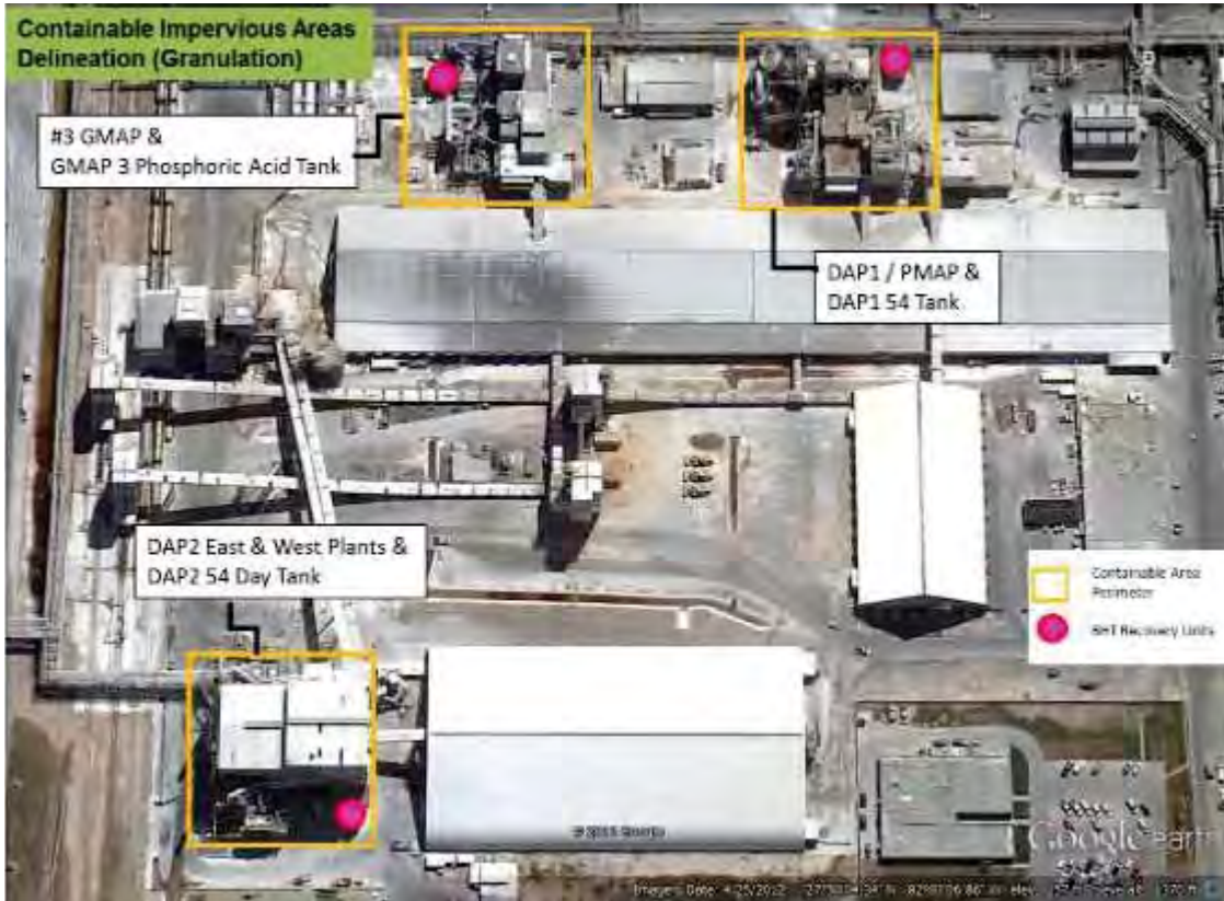
Figure 10: Containable Impervious Areas in Granulation
