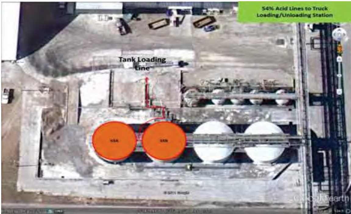
Figure 3: BHT Recovery Units - Downstream acid transfer lines from #4 DAP 55A Tank or 55B Tank to Truck Loading (see corresponding Table 2)
