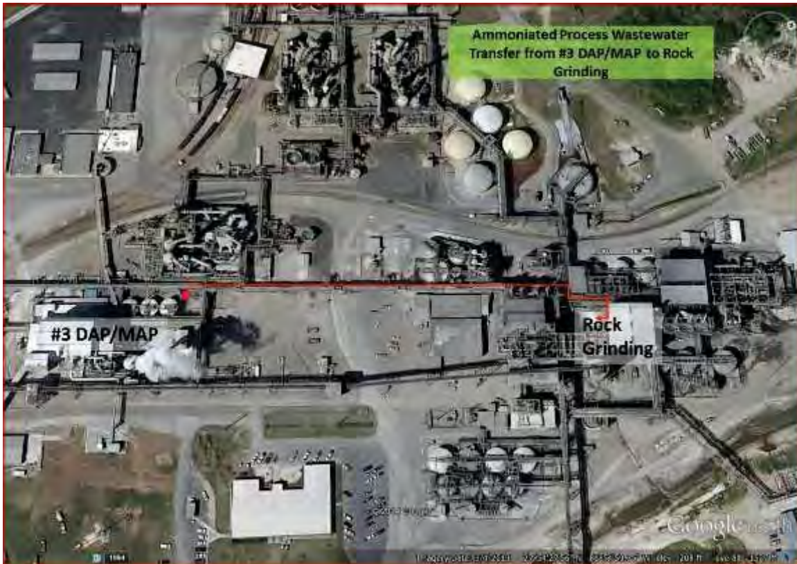
Figure 8: Ammoniated Process Wastewater Transfer from #3 MAP/DAP to Rock Grinding (corresponds with Table 6)
