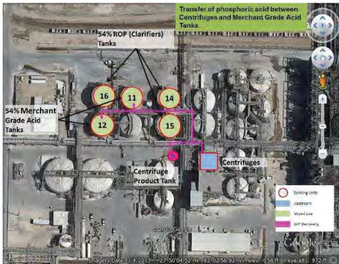
Figure 7: BHT Recovery Units for transfer of phosphoric acid between Centrifuge Product Tank and Merchant Grade Acid Tanks (corresponds with Table 7)
