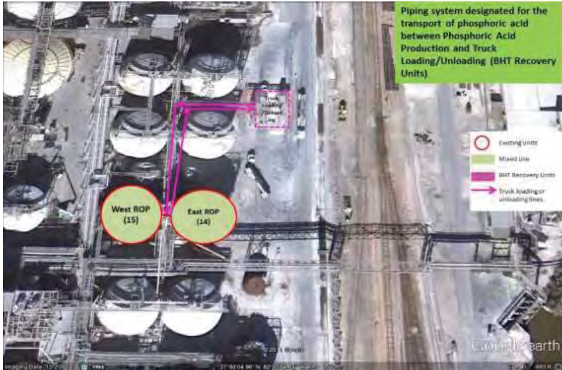
Figure 3: BHT Recovery Unit transfer of phosphoric acid between the Phosphoric Acid Plant and Truck Loading/Unloading (corresponds with Table 3)
