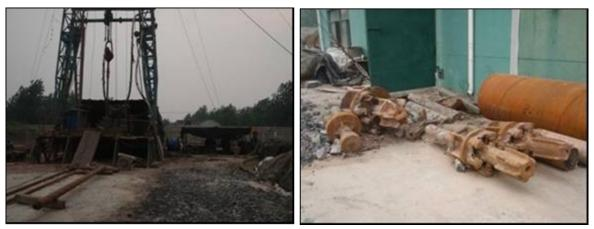
Figure 4-6: Surface to In-Seam Drilling Rig and Hole Opening Drill Bits
