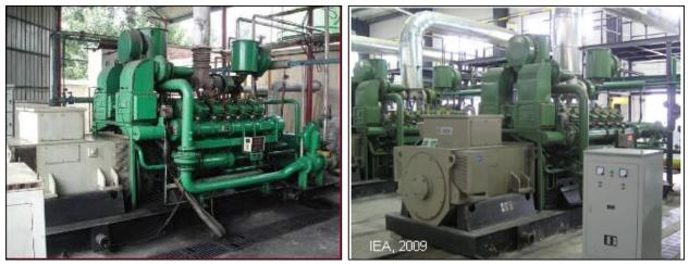
Figure 5-6: 500 kW Shengli Reciprocating Engine and Generator
