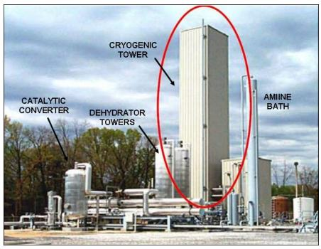
**Figure 5-7:** Cryogenic Gas Processing Plant (Jim Walters Resources mine in Alabama, U.S.) (Source: Katz, 2006)
