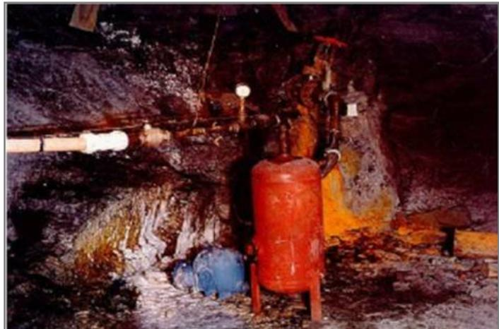
Exhibit 31: Separation system at the base of a vertical collection well
