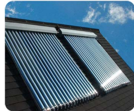
Solar Hot Water
