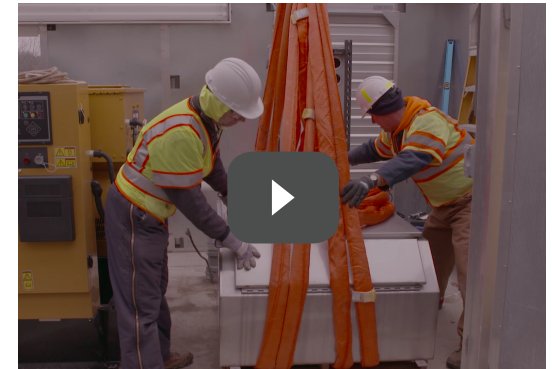
Video: Generator Placement
