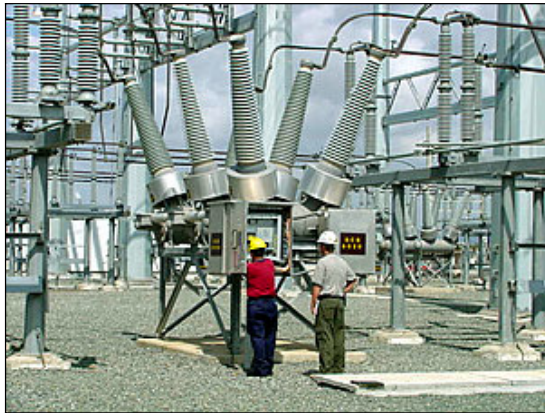
Fig. 1. Typical 245 kV dead tank circuit breakers using SF 6 gas as internal insulation and interrupting medium. This is Air Insulated Switchgear (AIS) as described later.
