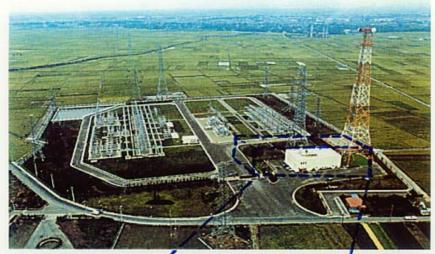
KITAKUMAGAYA, SUBSTATION(275kV)900 MVA) (An air-insulated-type openair substation)
