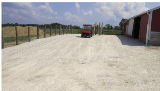
Figure 2. A farm's livestock loafing area, before (top) and after (bottom) a heavy-use area protection practice was installed. Photo by EPRI.
