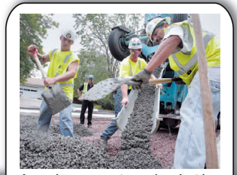
A pervious concrete road project in Minnesota attracts national attention. See article on page 14.
