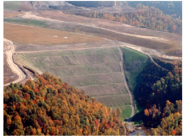
A mountain valley is completely filled with mining spoils from adjacent mining area. The site has been graded and planted with a ground cover.
