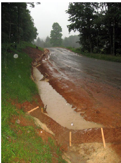
This photo shows a series of FCDs sprinkled with PAM successfully slowing runoff during a rainstorm at the study site.
