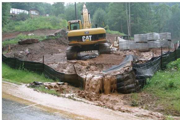
The erosion control practices on this construction site are poorly designed and maintained, which allows excessive sediment to be carried off-site during heavy rainfall events.
