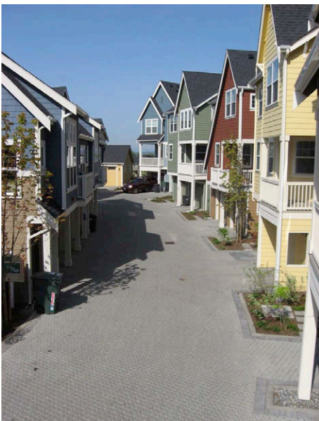
This Seattle town home development uses pervious pavers in alleyways to reduce runoff. The goal of the Local Regulations Assistance Project is to facilitate low impact development projects such as this throughout the Puget Sound region.
