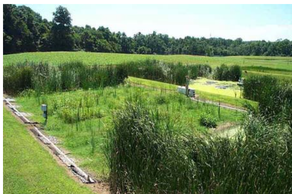
Two of the research facility's four wetland treatment cells are shown here.
