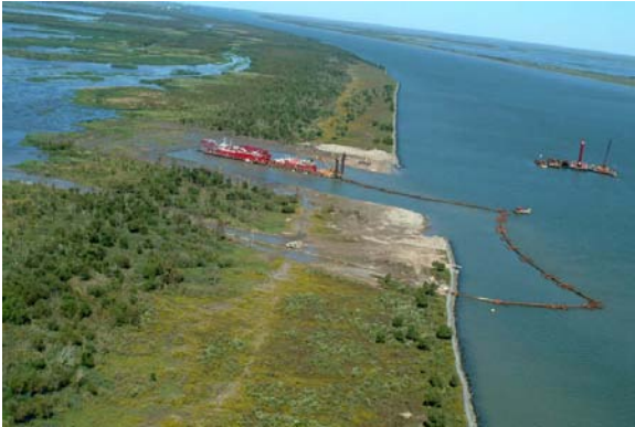
As a diversion is dredged from the Mississippi River (on the right) to the West Bay, the sediment slurry is pumped through pipes to the West Bay restoration site (Photo credit: U.S. Army Corps of Engineers New Orleans District).
