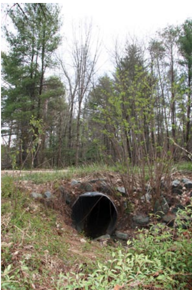
This culvert protects a small stream from logging traffic above.
