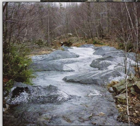
Examples of the open limestone channels (left) and diversion wells (above) built to help treat acid mine drainage in the Swatara Creek watershed.
