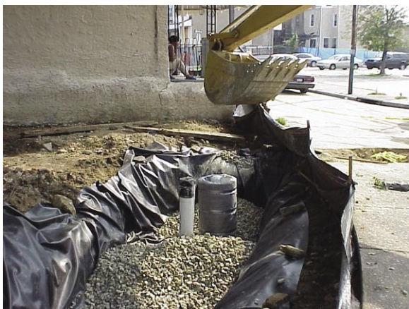
LID pocket park under construction.
