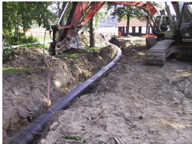
The pipe was buried underground from the lake to the discharge point.
