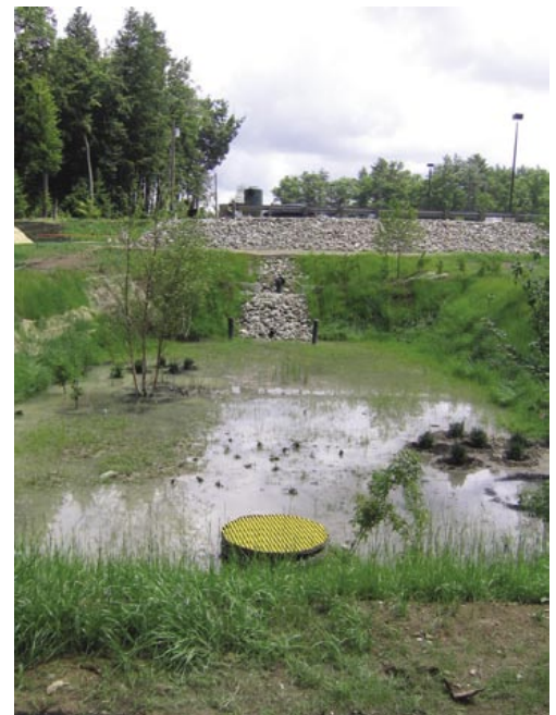
This bioretention unit is one of the low-impact development systems currently being tested at CSTEVE.
