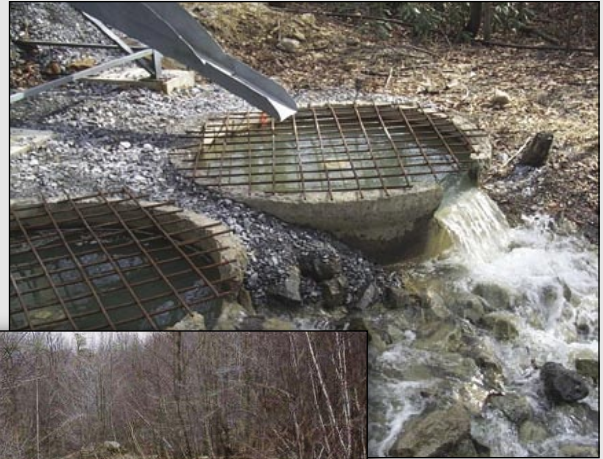
Examples of the open limestone channels (left) and diversion wells (above) built to help treat acid mine drainage in the Swatara Creek watershed.
