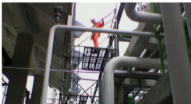
PEMEX engineer descends scaffold tower after taking wet seal measurements at a PEMEX gas processing center.
