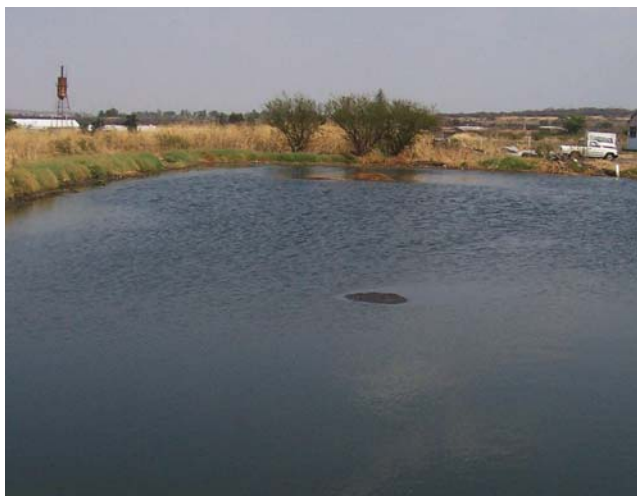
Anaerobic digester effluent lagoons are used in many confined animal operations for stabilization and temporary storage of manure wastes. This lagoon is located at the Santa Monica Farm in La Piedad, Michoacán, Mexico.
