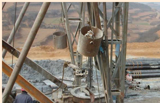
Construction of the world's largest CMM-generated power project (120 MW capacity) at Sihe Mine, Jincheng, Shanxi Province, China.
