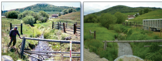
Figure 2. A site in the Upper Rapid Creek watershed, before (left, 2001) and after (right, 2007) BMPs were installed to protect the stream corridor and reduce erosion.
