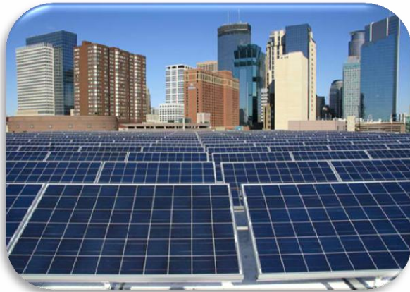
Solar rooftop or Ground-mounted near facility
