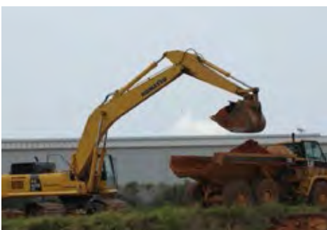
Removal of the last part of “Mt. Dioxin,” a huge pile of contaminated soil at the Escambia Wood Treating Company site.
