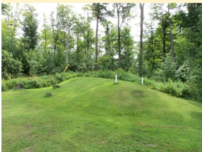
Mounded wastewater treatment system for a Lac Vieux Desert Band home
