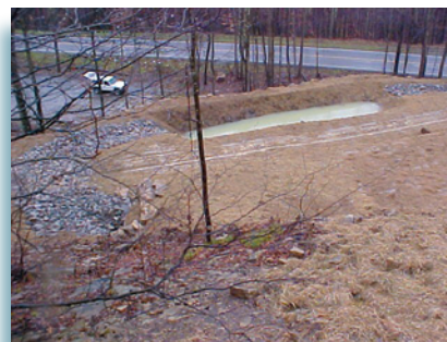
View of outlet from anoxic limestone drain through the short open limestone channel and into the settling basin.
