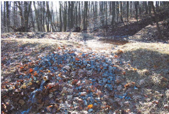
Limestone leach bed and outflow soon after completion in fall 2003.
