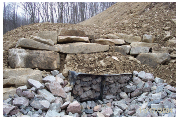
Trap design using stone in wire mesh baskets to help aerate the water. It then flows through the short open limestone channel into the settling basin.
