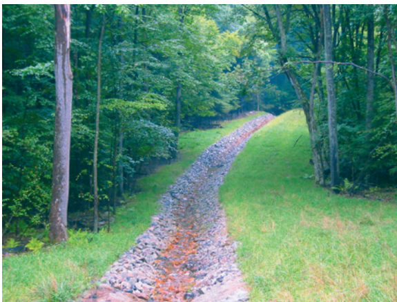
Open limestone channel running through the woods with coloration starting to show iron precipitate.
