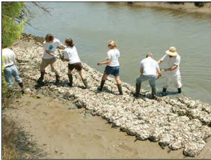
Figure 3. Partners pass mesh bags of oyster shells as they help to create an oyster reef on Tibwin Creek.
