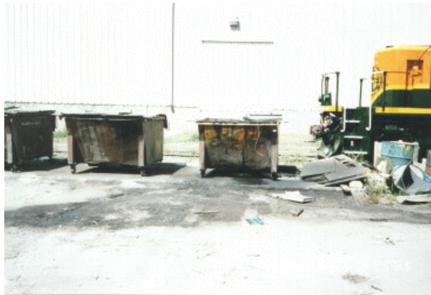
The MT27 facility. The dark area in the concrete represents used oil contamination.
