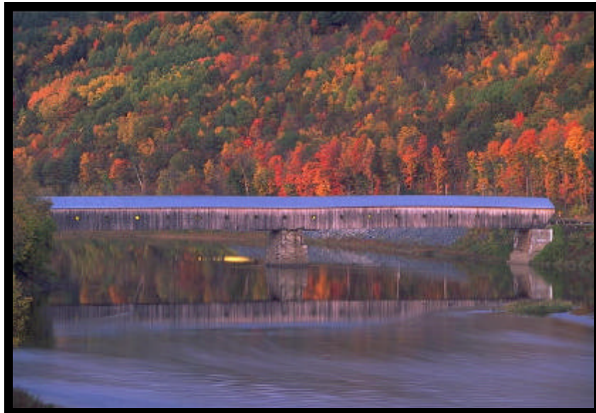
Windsor-Cornish Bridge, Cornish, New Hampshire
