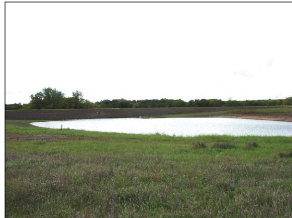
Figure 1. One of several water quality basins constructed in the watershed to complement land treatment measures. These basins are effective at controlling steep grades and trapping pollutants that are mobilized during larger storm events. Each structure is fenced to exclude livestock and alternate livestock water is provided below the structure.
