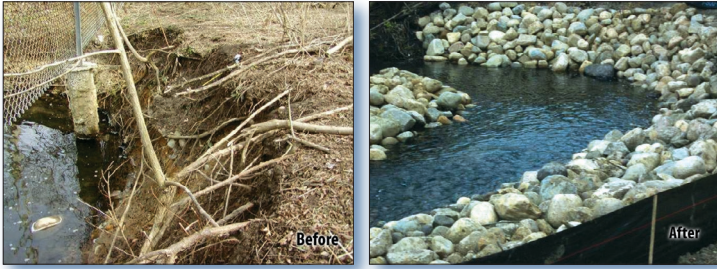
Figure 2. Project partners reshaped the streambank and added rock to stabilize this eroding area of Arcadia Creek along Stadium Drive on the Western Michigan University campus.
