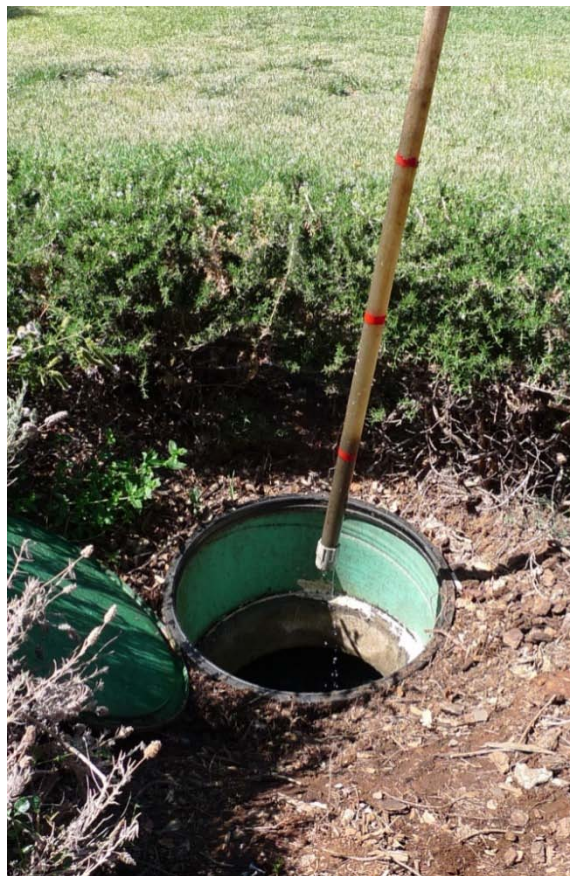
Figure 3-9. Sludge Measurement Taken at Site 4. The Red Marks are Located Every Foot.
