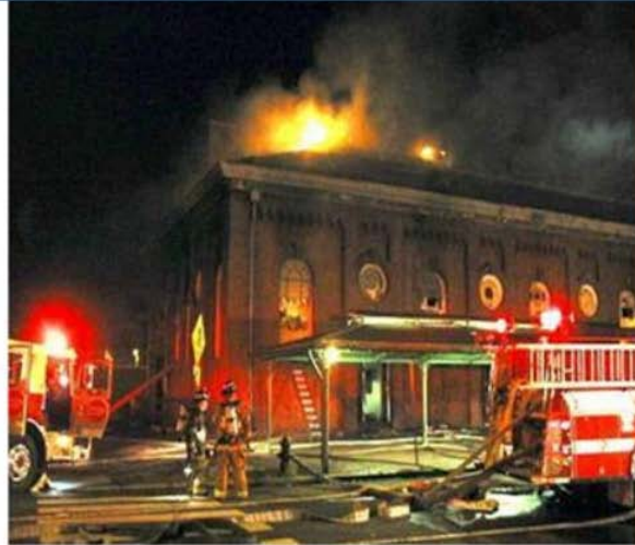
Fire at DC's historic Eastern Market Credit: Arthur Delaney, Washington City Paper
