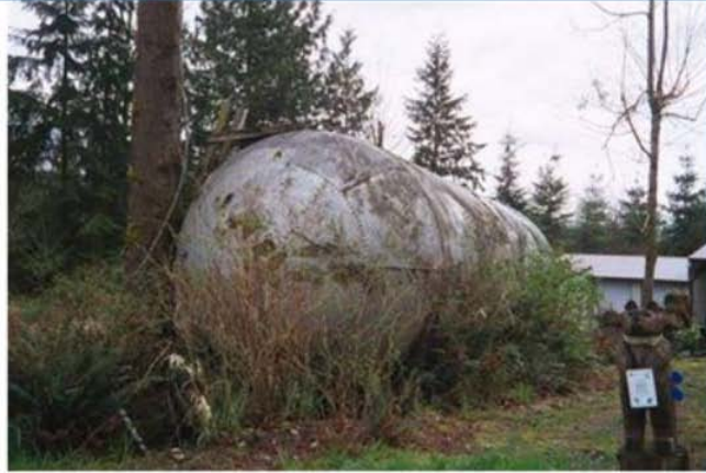
Poorly maintained reservoir
