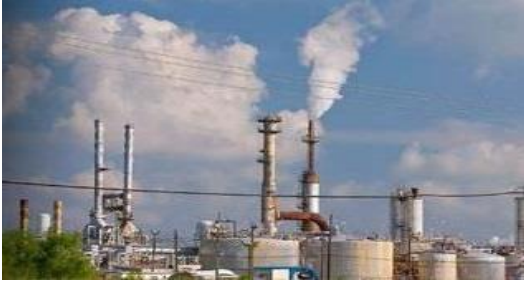
A sulfuric acid plant. (EPA photo)
