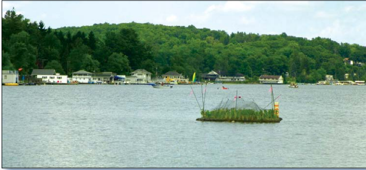
Figure 2. Watershed partners reduced the in-lake total phosphorus of Harveys Lake by installing floating wetland islands that absorb nutrients from the water.
