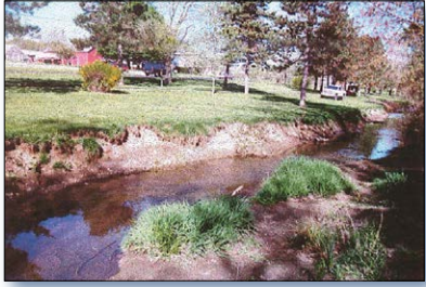
Figure 2. In 2001, partners addressed an eroding, incised section of Bear Brook in East Windsor Township's Anker Park (as seen on left, March 2001) by implementing bioengineering and revegetation riparian restoration techniques (as seen in the middle, May 2001). By July 2014 (as seen on right), Bear Brook had a healthy, well-established riparian buffer that provides shade and protects against erosion.
