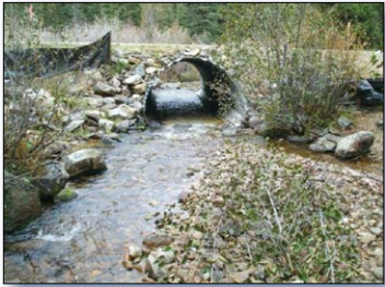
Figure 3. Partners replaced a forest road culvert (left) with a new bridge (right) over Meadow Creek. The bridge allows unimpeded fish passage and reduces road-related sediment loads.
