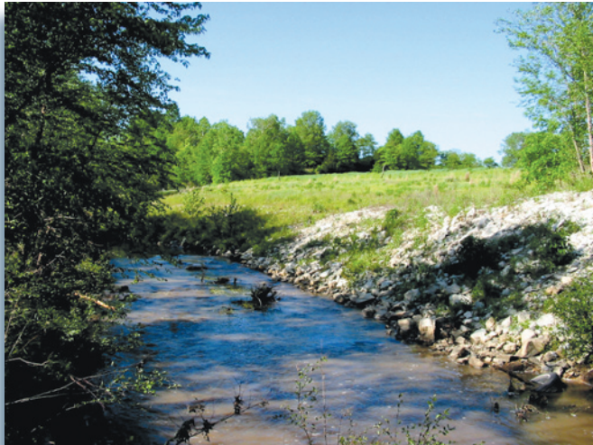
Native trees and grasses are thriving along sections of restored streambank.
