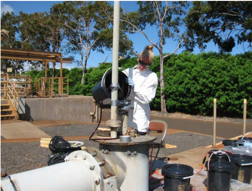
Figure 4-8: The residual dye was poured directly into the well.
