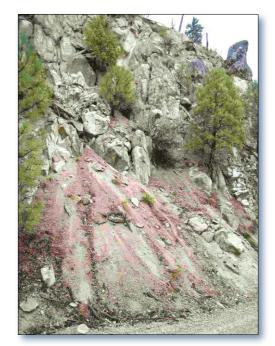
Figure 2. An eroding road cut in the South Fork Payette subbasin (photo by USDA Forest Service).
