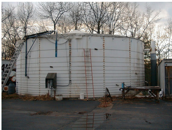
Figure 9.4. Above ground manure storage structure
