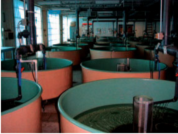
Figure 3.2. A recirculating system
