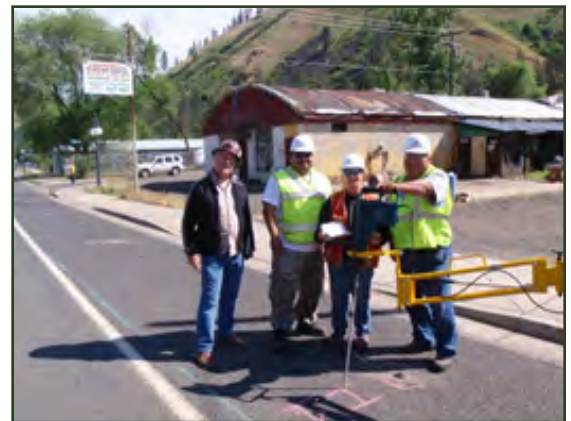
Groundwater Program installing soil vapor sampler.
