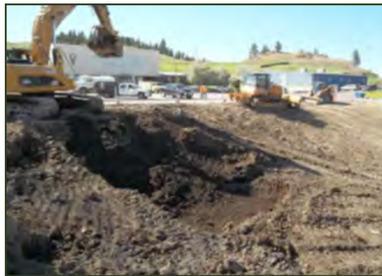
Excavation of a fuel contaminated hillside near Sundance Creek.
