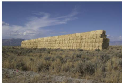
Fig. 1. Mock-up of hay bales barrier, 6 m high and 100 m long. Finn et al., (2010)
