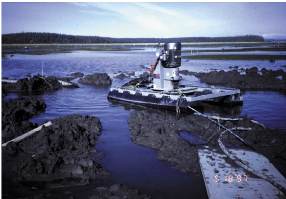
Figure 1. The Army placed pumping systems such as this one into the marsh to drain the water and allow the white phosphorus to oxidize into a harmless state. For more images of the restoration project, see www.crrel.usace.army.mil/erf/photographs/photos-remediation .
