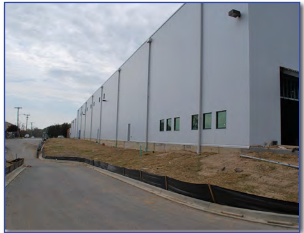
After: New Facility
