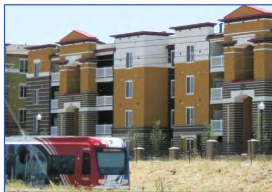
Former Simpson Steel Site - After
