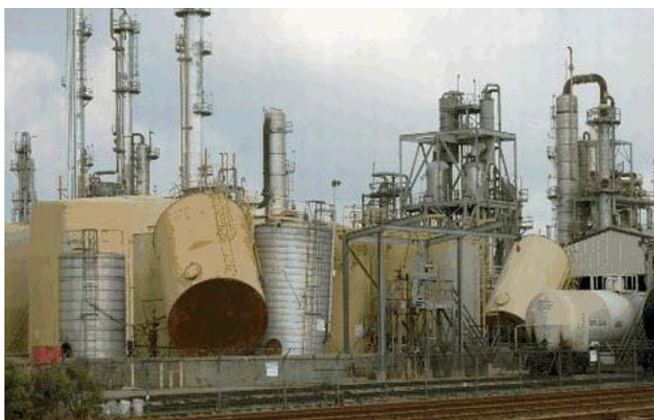
Figure 2- A chemical manufacturing facility in Mississippi after the hurricane. (Source: EPA)
