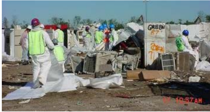
Figure 10 – EPA contractors removing contents and recycling Freon from refrigerators at Old Gentilly landfill in Louisiana. (Source: EPA OIG)
