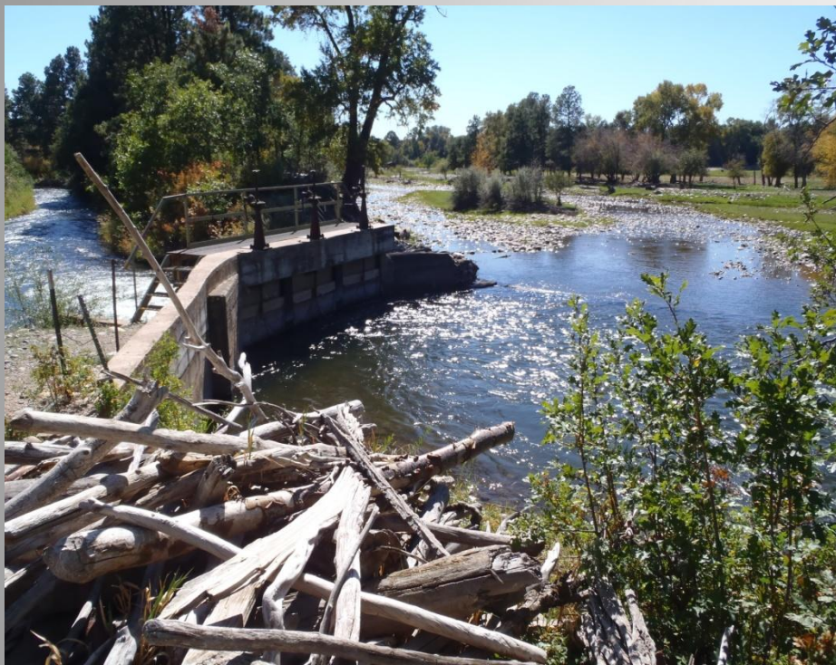
Pine Ditch Diversion
